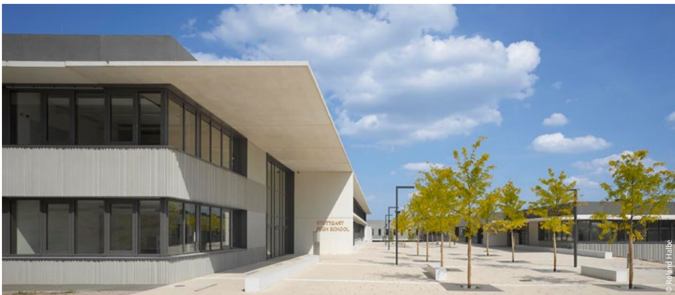
American High School & Elementary School, Stuttgart-Böblingen
